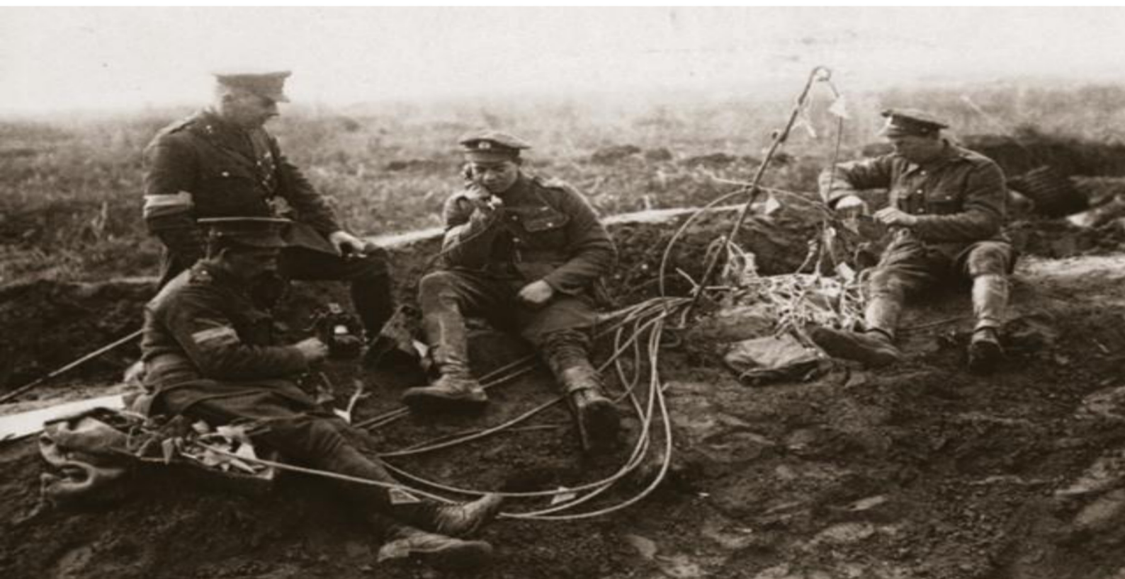
Royal Engineers instalando linhas telefónicas (Flandres, 1917)
